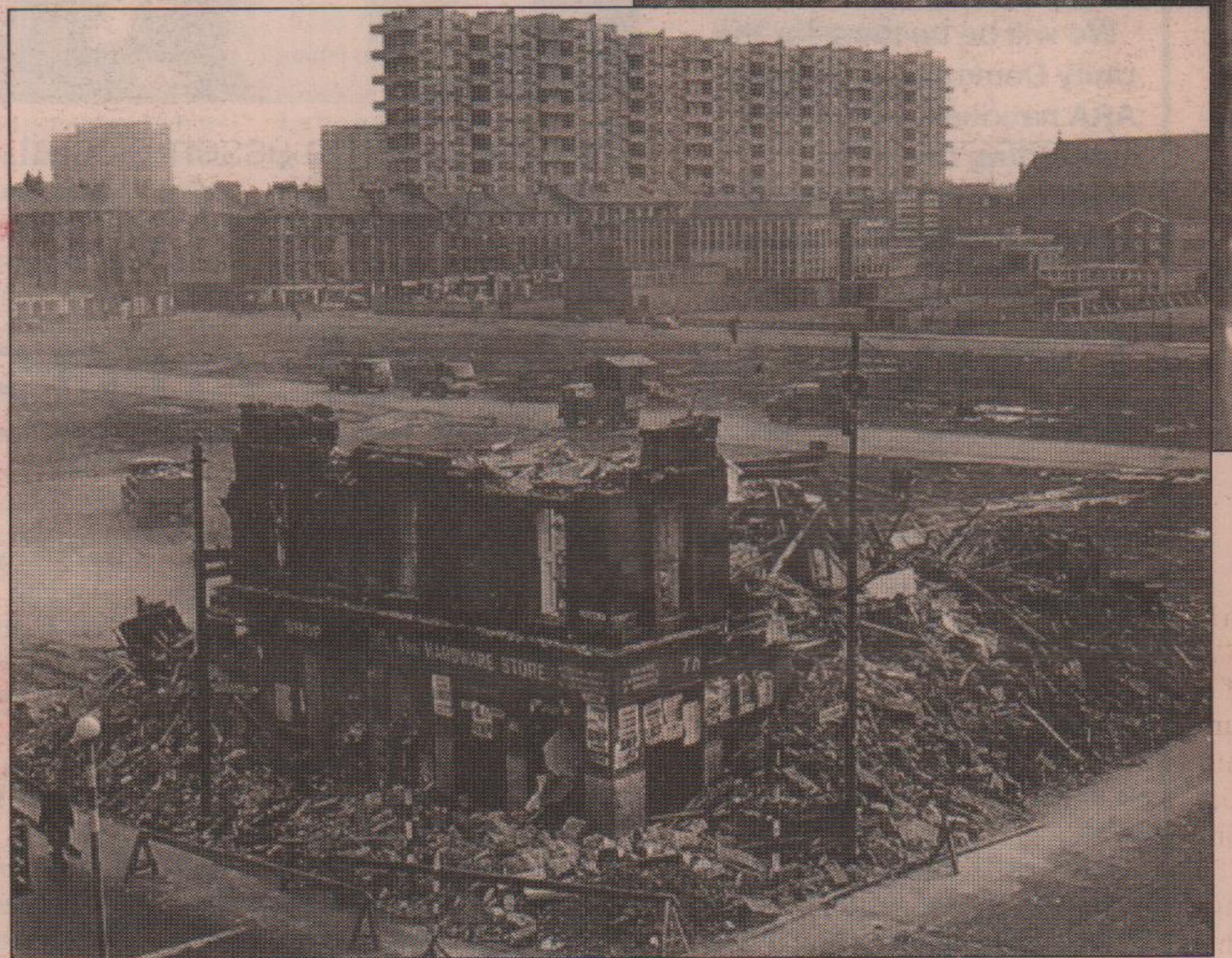
Queen Elizabeth flats under construction
